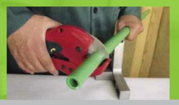
For successful joining of pipes, at least three preparation stages must be followed:
